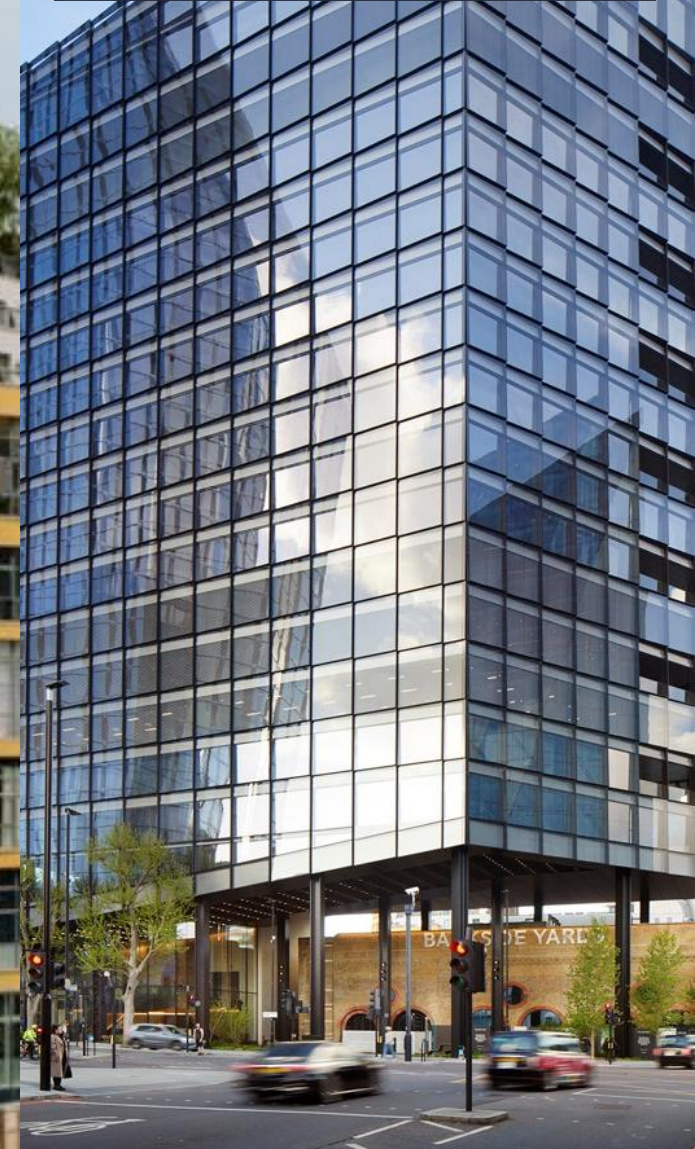
ARBOR TOWER, BANKSIDE YARD (DEFENDANTS)
